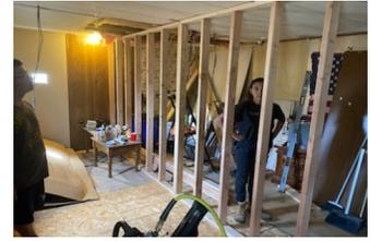
We were able to replace the floor and the ceiling in one area to prevent animals from coming in. We then demolished a wall and rebuilt a wall dividing the room into 2 separate rooms.
